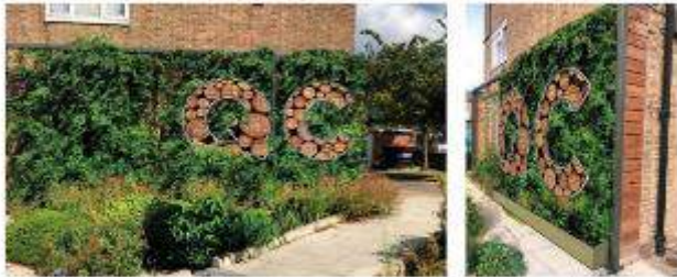
SuDSPlanters Living wall 24 m² area - 15 plants and 100 litres water Proven 1 SuDS - 800 litres rainwater
